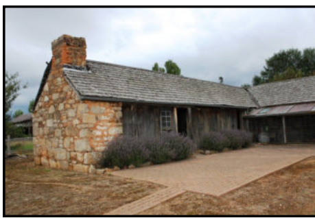
Rear of Settler's Cottage
